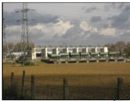
Tail Sluice - One of the biggest pieces of flood risk infrastructure in the country. Part of Ely Ouse Flood Protections Scheme. Allows discharge from Relief Channel at low tide.
