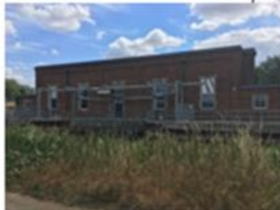
Welches Dam Pumping Station - pumps water from the Counter Drain when gravity discharge not possible.
