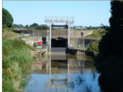
Old Bedford Sluice - water from Counter Drain can discharge at low tide.
